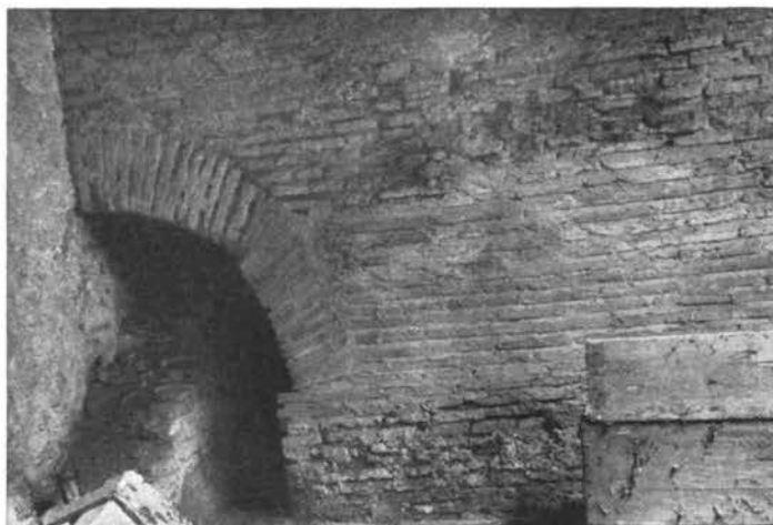
Fig. 232 — S. Maria in Cosmedin. exterior of north wall of left aisle; remains of earlier niche (Photo: Corbett).
